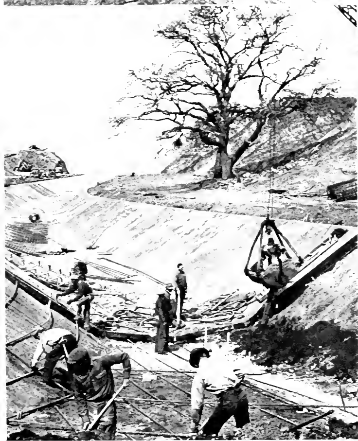
Top picture shows completed portion of flume, paralleling Grapevine Grade highway, for carrying creek waters past side area. Lower pictures show work on reinforced concrete lining of flume and the special spillway construction at its lower end.
